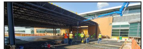
Finishing the concrete for the south bridge deck in early August
